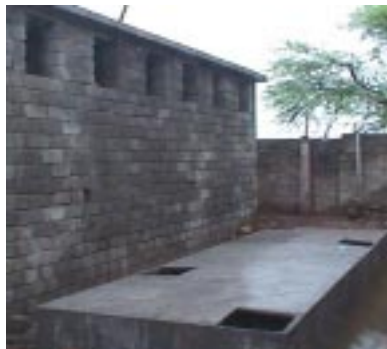
Block walls and the ferro-cement tank at Sangam Wadi
