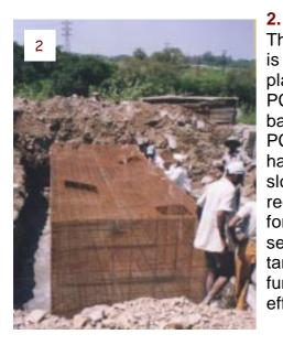
The cage is put in place on a PCC base. The PCC base has the slope required for the septic tank to function efficiently.
