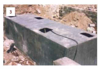
Every day the tank is filled with 6" of water to cure it from inside and to uncover any leaks in the tank walls.
