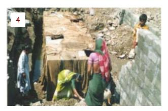
**4.** The outside of the tank is cured by placing wet gunny sacks over it. Here the women are lending a hand in filling the area around the tank.
