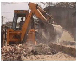
The JCB smashes the slab at Sangam Wadi: in half a day the tank was completely demolished
