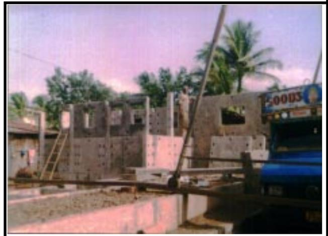
Hoisting prefab panels, columns and beams using cranes in Sangliwadi.
