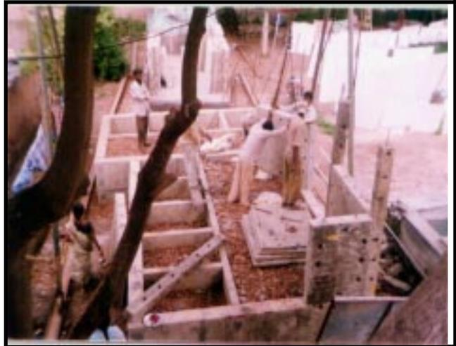
Assembling the precast wall panels of individual stalls in Tasgaon Ves
