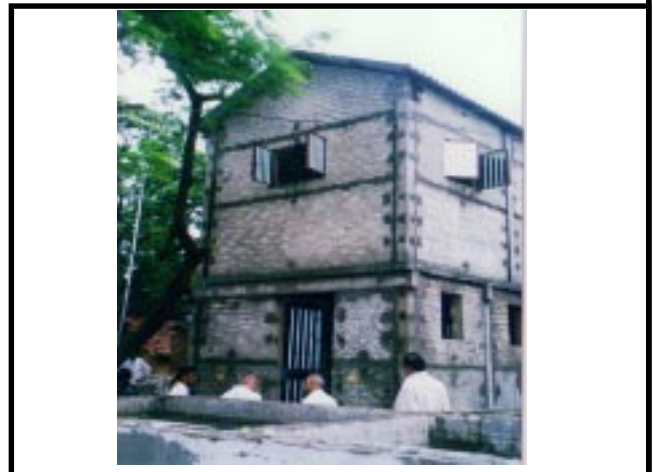
The Fully assembled toilet block at Tasgaon Ves.
