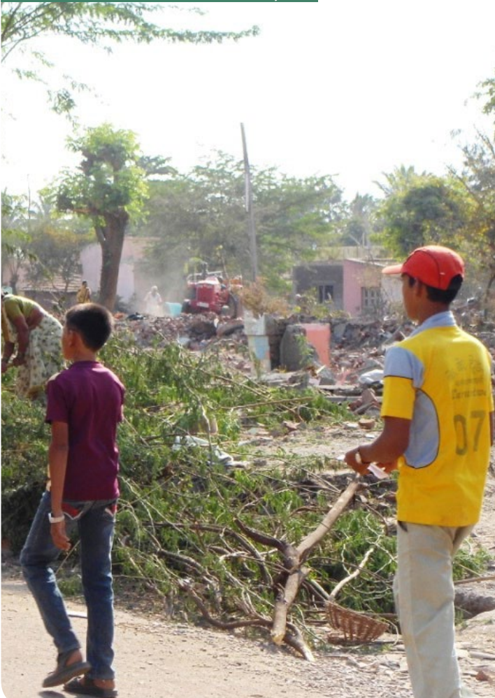
Demolishment went smoothly
