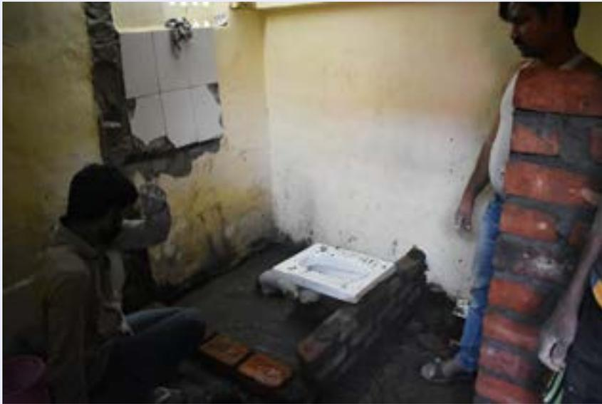
Fig 6. Building of the toilet, using brick masonry.
