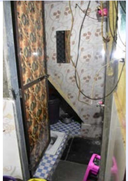
Fig 22. Toilet that has a staircase cutting through at House No. 416 at Vijay Nagar, Thane
