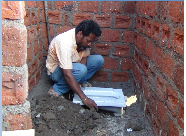
The orissa pan, p-trap and plumbing is installed
