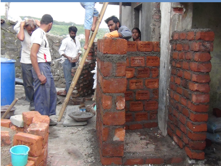
The external envelope being formed in brick and mortar
