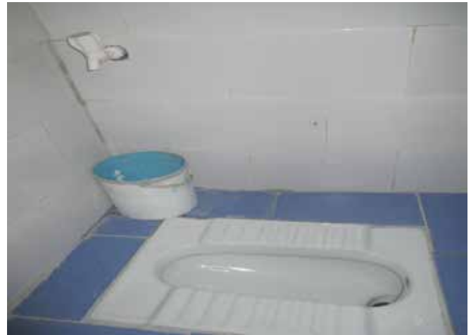
An “individual household toilet “built by Shelter Associates
