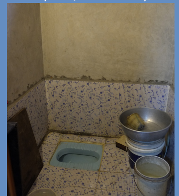
Example of toilet
