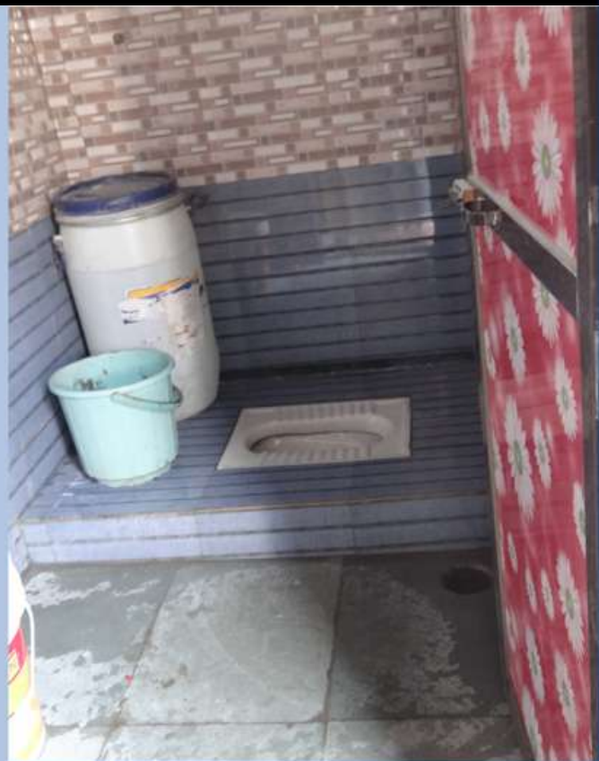
Toilet after construction.
