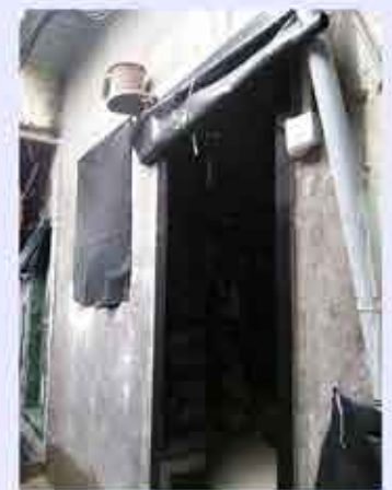
House being upgraded
