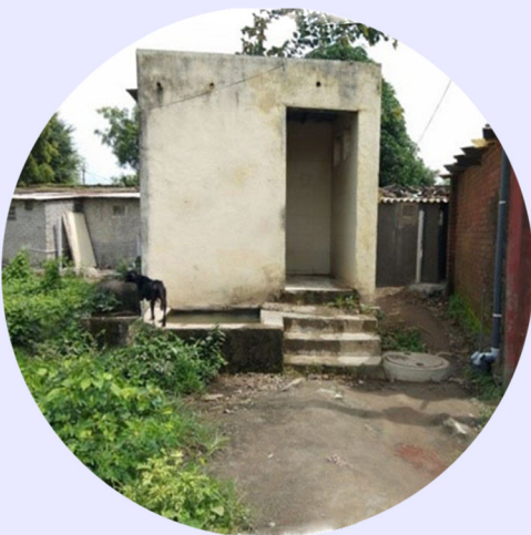
COMMUNITY TOILET BLOCK (CTB)
