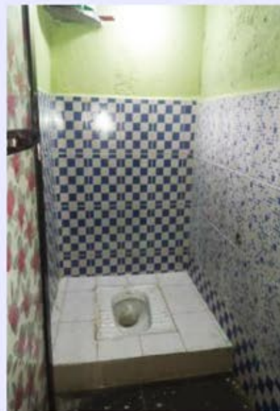
Vinayak's constructed toilet
