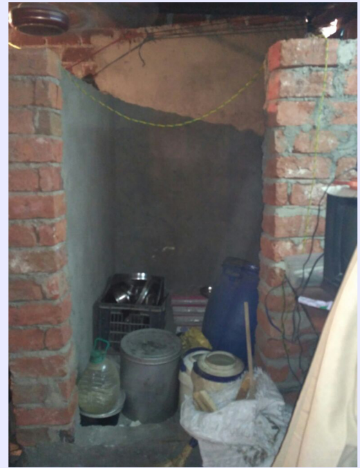
Ongoing toilet construction
