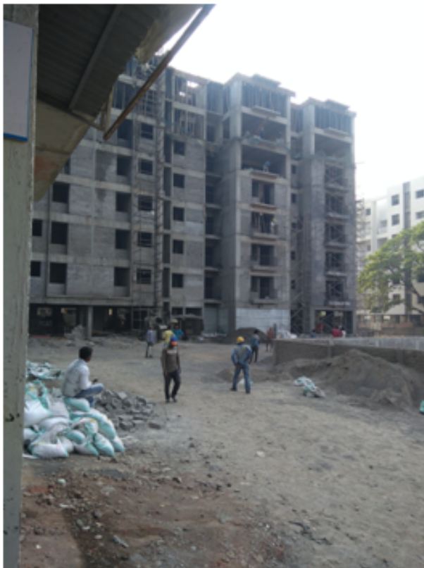
Figure. 4.7 View of Loknagari under construction building
