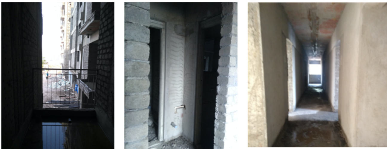
Figure. 4.9 View of Loknagari under construction building
