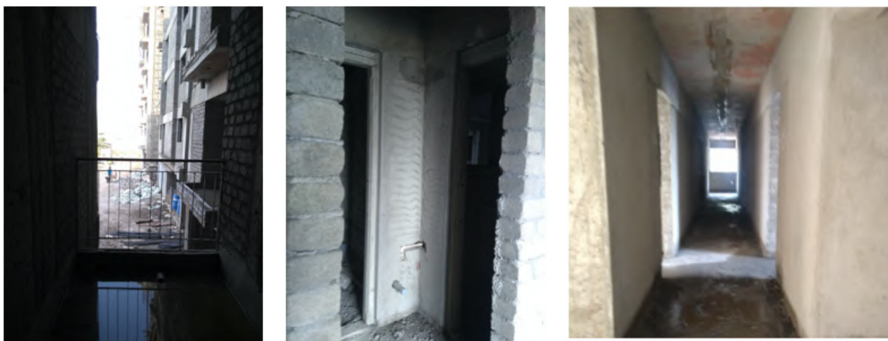
Figure. 4.9 View of Loknagari under construction building
