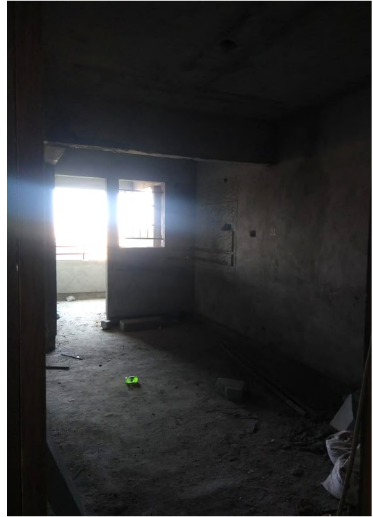
Figures. 4.6 Pictures of ongoing construction
