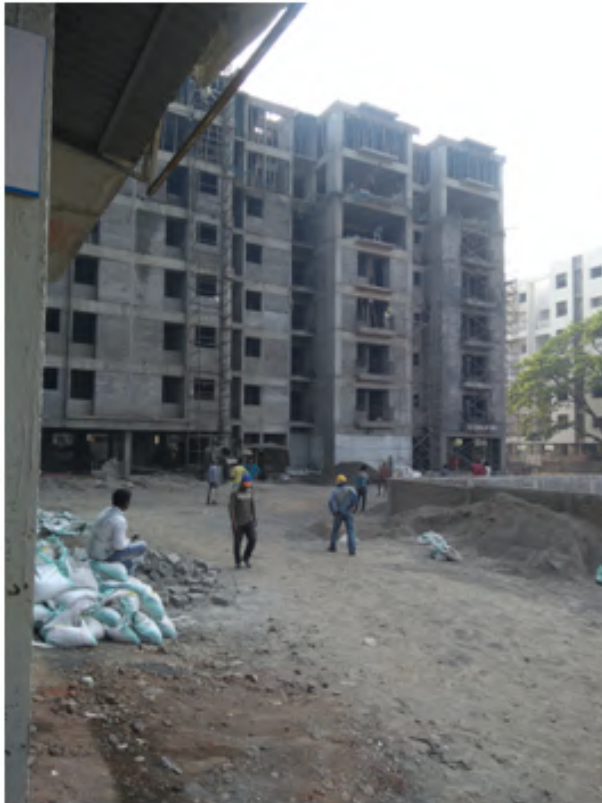
Figure. 4.7 View of Loknagari under construction building
