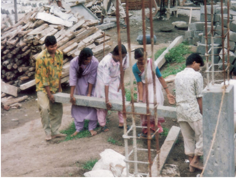
Fig. 5.2 Community involved in constructing their own houses at Dattawadi
